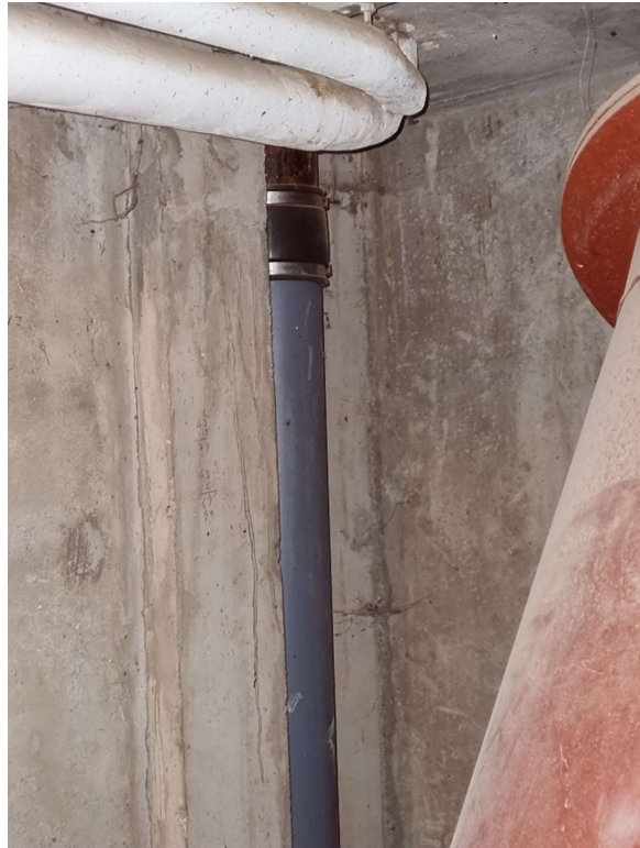
Drain pipe replaced because of leakage
